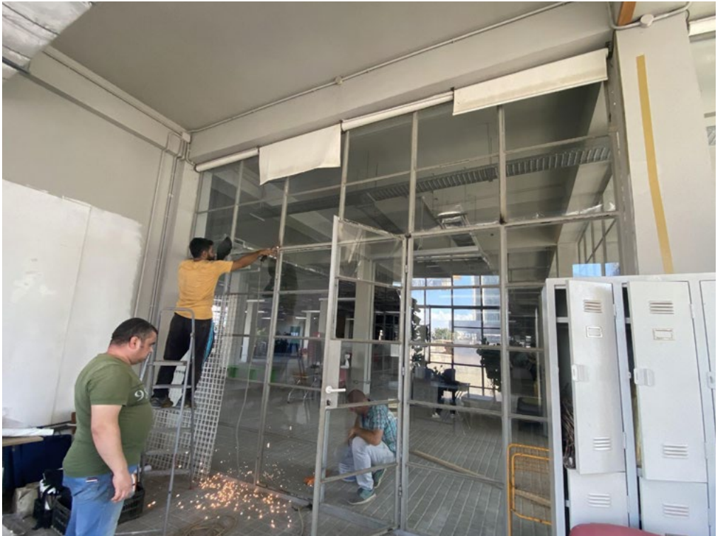
Repairs taking place at the Lebanese Association for Plastic Arts, Ashkal Alwan
